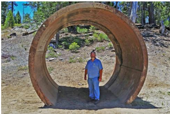
Section of Penstock Pipe
