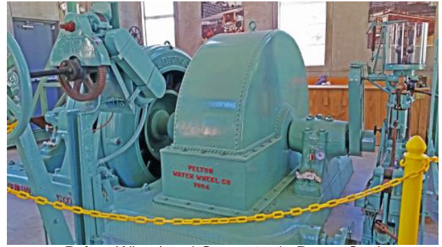
Pelton Wheel and Generator in Power Station
