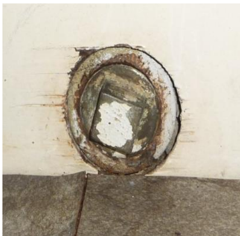
Old Drain Clean-out Plug
