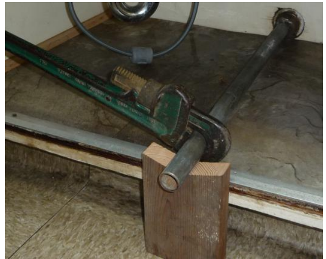
Final Setup W/ Socket, Pipe Wrench and Support Block
