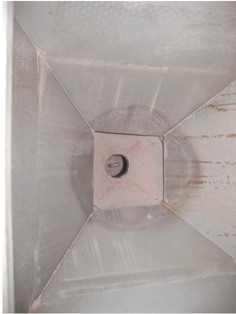
View down into Hopper after Modifications
